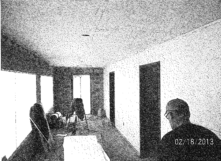
#3--Setting drywall on the 2nd floor of the Press Box.
